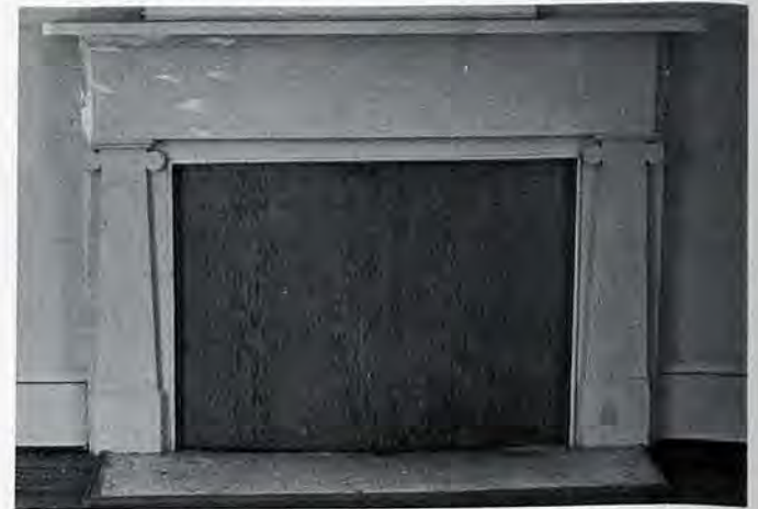
Figure 14. Vernacular Greek mantel. A simple post-and-lintel composition, with knobs at the tops of the pilasters representing the volutes of the capitals of the Ionic order.
