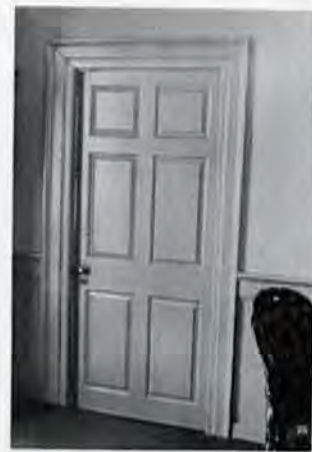
Figure 7. Georgian-type door. Six raised panels in a three-part surround.
