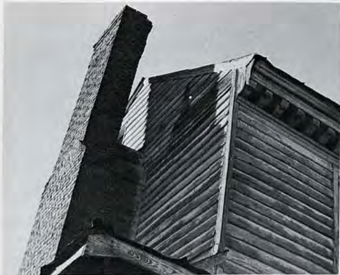
Figure 6. Georgian-type cornice. The cornice is boxed, and here treated with ornamental modillion blocks. The sawn pattern board at the end is a cross-section of the cornice and its moldings. The roof is flush with the gable end. Note the free-standing stack of the chimney.
