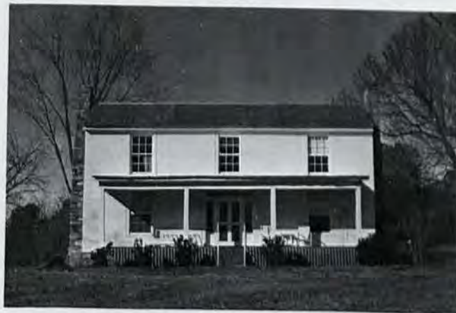
Figure 12. Marcus Carpenter House, Franklin County. A simpler gable-roof mid-nineteenth century house with Greek moldings. Compare facade with Figures 2,3,4, and 9. This house is now covered with asbestos siding.
