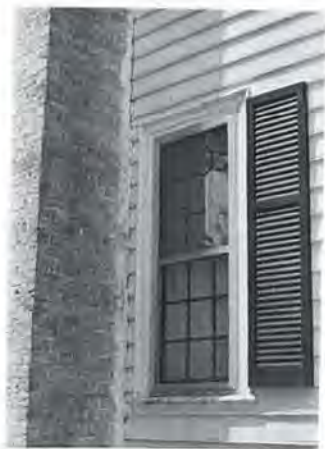
Figure 5. Georgian-type window. Nine-over-nine sash, three-part molded and mitred frame, and molded window sill. Note beaded weatherboard.
