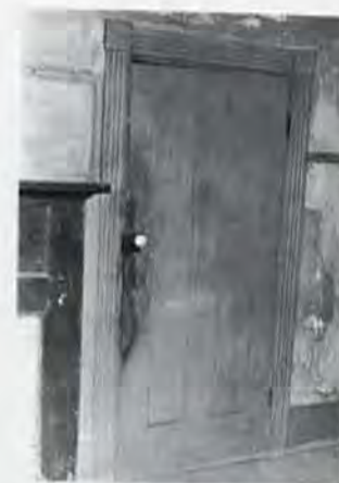
Figure 13. Greek Revival-type door. Two long vertical panels. The door frame is symmetrically molded with square blocks set in the upper corners. This same type of frame also appears around exterior doors and windows.
