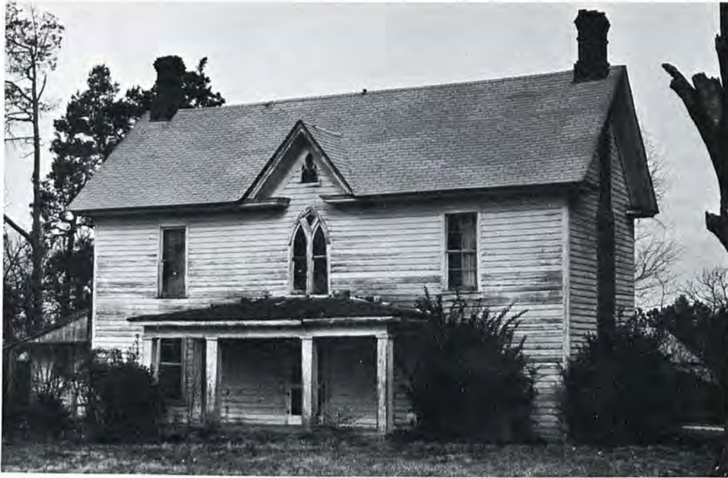
Figure 16. Benjamin Wyche House, Vance County, ca. 1870. An I-house with a specific reference to the Gothic Revival with the pointed-arch second story central window. The center gable, in various forms, becomes a common feature of later nineteenth century houses (Figures 1 and 17).
