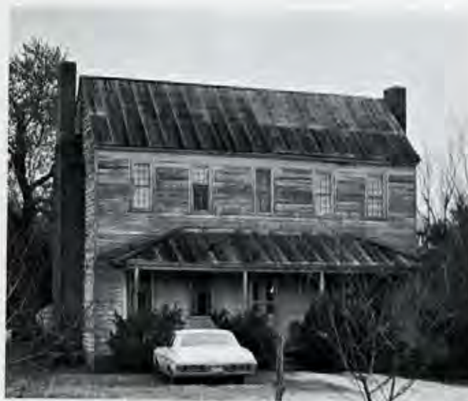
Figure 2. Foster House, Franklin County, late eighteenth century. This house has the symmetrical five-bay facade associated with formal Georgian architecture. Note the tall, narrow windows with nine-over-nine double-hung sash (the first floor sash has been replaced). The roof is flush with the gable ends. The porch here is not original; early porches have rarely survived.
