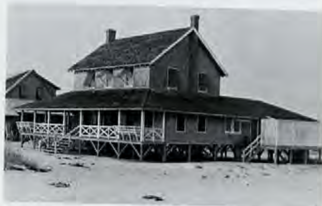
Figure 6. A simple gable-roof two-story cottage at Nags Head Beach.
