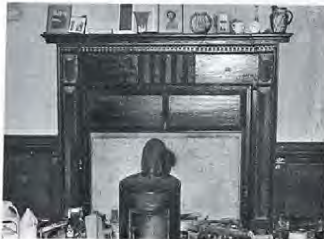
Figure 10. Federal mantel. Flat surfaces and delicate reeding and carving. This is the "three-part" format with a center plate here reeded in a herringbone pattern.
