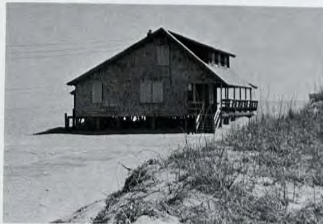
Figure 14. A new cottage incorporating many of the traditional cottage features.
