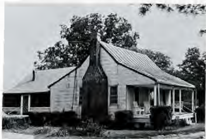
Figure 15. Duplin County "coastal cottage" type hall-and-parlor house.
