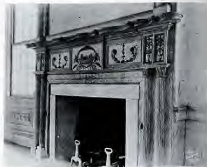
Figure 3. Montmorenci, drawing room mantel, in situ . The elaborate decoration, of molded composition material, is thought to be the work of Philadelphia ornament manufacturer Robert Wellford. The central panel is decorated with a scene of the Battle of Lake Erie (1814). The carved rosettes and garlands around the fire opening are similar to patterns found in other related houses.
