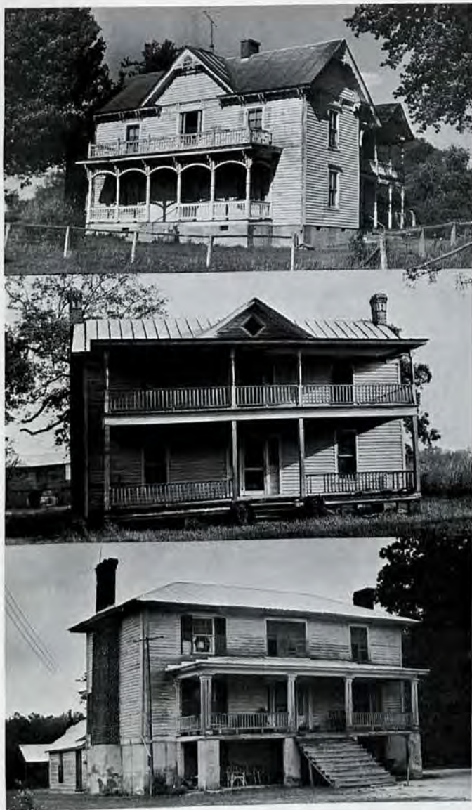
Figure 25. Three North Carolina central-hallway I-houses, (from top down) in Ashe, Duplin, and Granville Counties.
