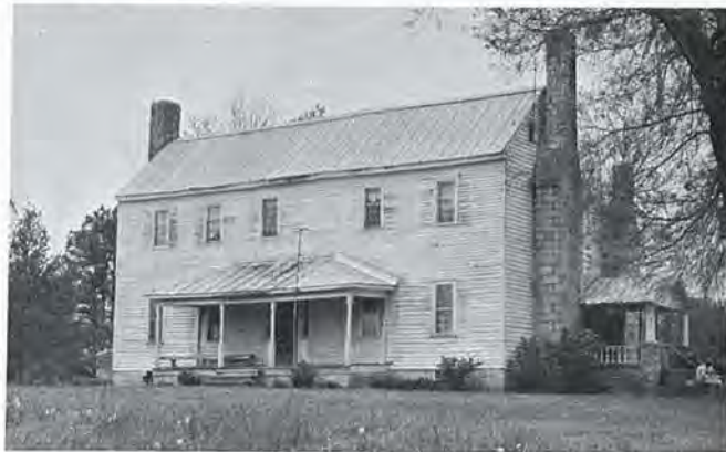
Figure 4. Young House, Vance County, early nineteenth century. This is probably the largest early I-house surviving in the region. In the mid-nineteenth century it received a two-story rear shed addition, making it a double-pile house. The exterior is in the Georgian tradition and has the "Georgian symmetry" except for the placement of the second-story central window. The interior is a curious blend of Georgian and Federal elements with Greek Revival touches dating from the time of the rear addition.
