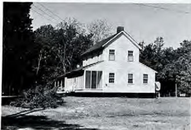
Figure 4. A familiar rural North Carolina house type at Kitty Hawk Village.
