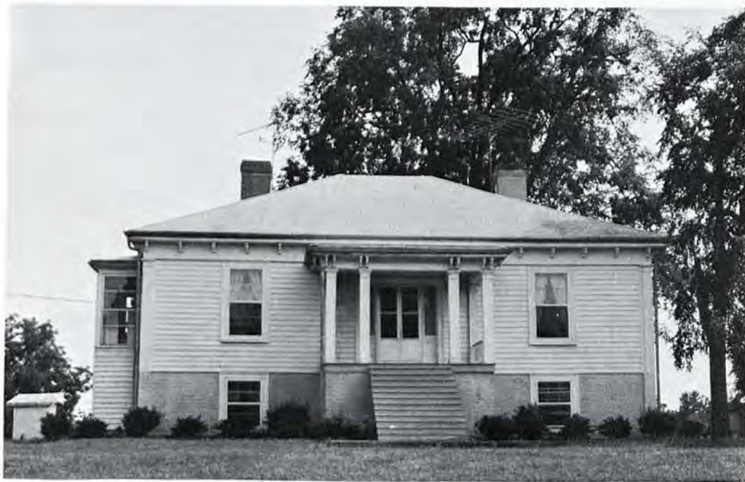
Figure 22. One-story Georgian-plan house in Franklin County on a raised foundation and with Italianate and Greek Revival decorative elements.
