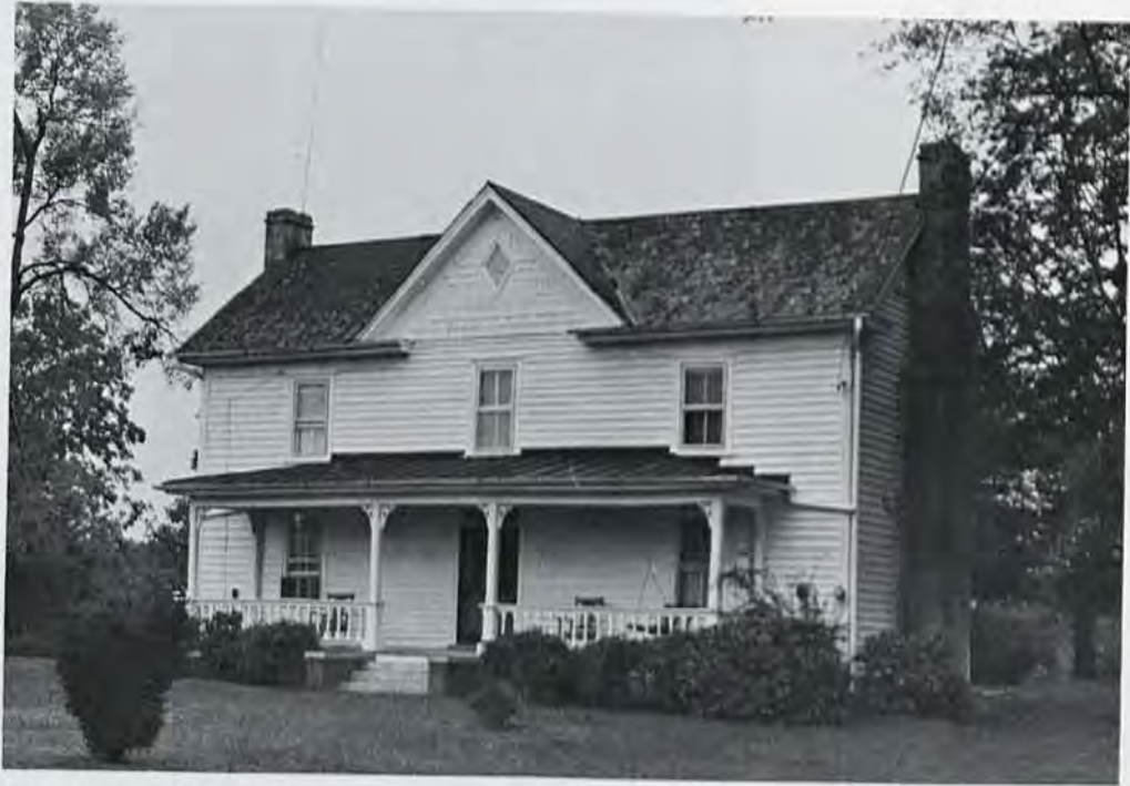
Figure 1. Floyd-Morris House, Granville County. This I-house has the center gable, here with shingle ornament, typical of many houses built in the region in the late nineteenth century. The chimney is dated 1896.
