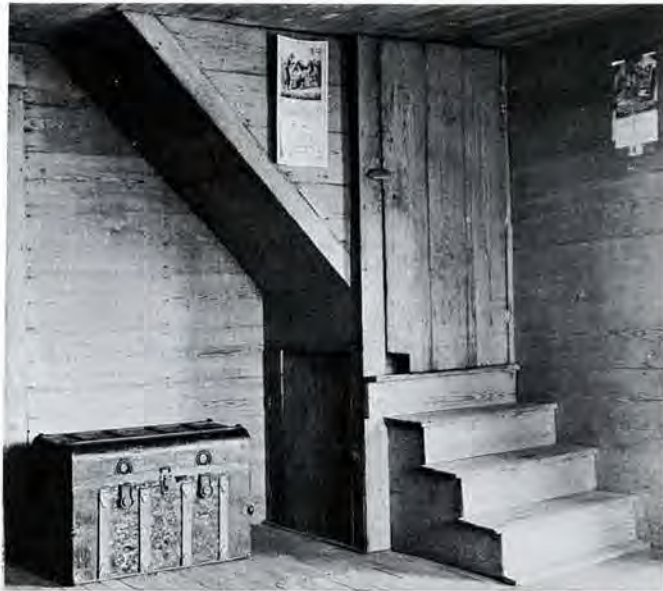
Figure 10. Boxed-in stairway in an eastern North Carolina tenant house.
