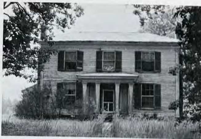
Figure 11. Terrell House, Franklin County. This is a good example of the Greek Revival in this region, showing the changes in proportions. The three-bay facade has large, squarish windows of six-over-six sash. The house is covered in a low-pitched hip roof. The facade is framed with wide corner posts, here fluted, and the wide frieze under the cornice is given a Greek key ornament. The porch, which is original, duplicates these ornamental features.
