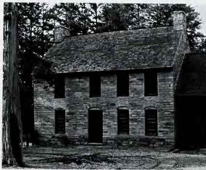
Figure 13. The Michael Braun House, or “Old Stone House,” in Rowan County, built around 1770.
