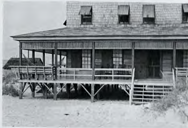
Figure 10. Wooden batten window shutters function as shades as well.
