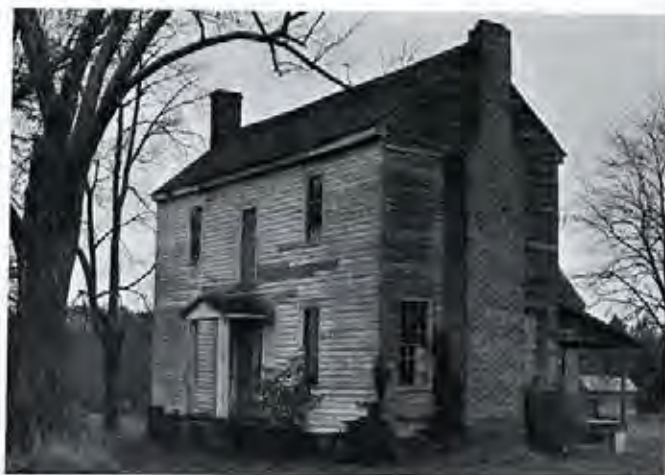
Figure 9. Mitchell House, Franklin County, ca. 1820. The exterior form of this house differs little from its predecessors. It originally had a two-tiered porch. Window sills are unmolded. Note the mass of the chimney and its concave shoulders; compare with the chimney of Figure 3.
