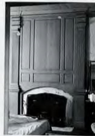
Figure 8. Georgian mantel. Bold composition of raised panels over an arched fire opening.
