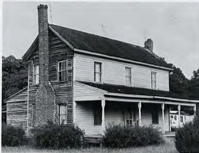
Figure 20. Front view of the same Duplin County central-hallway I-house.
