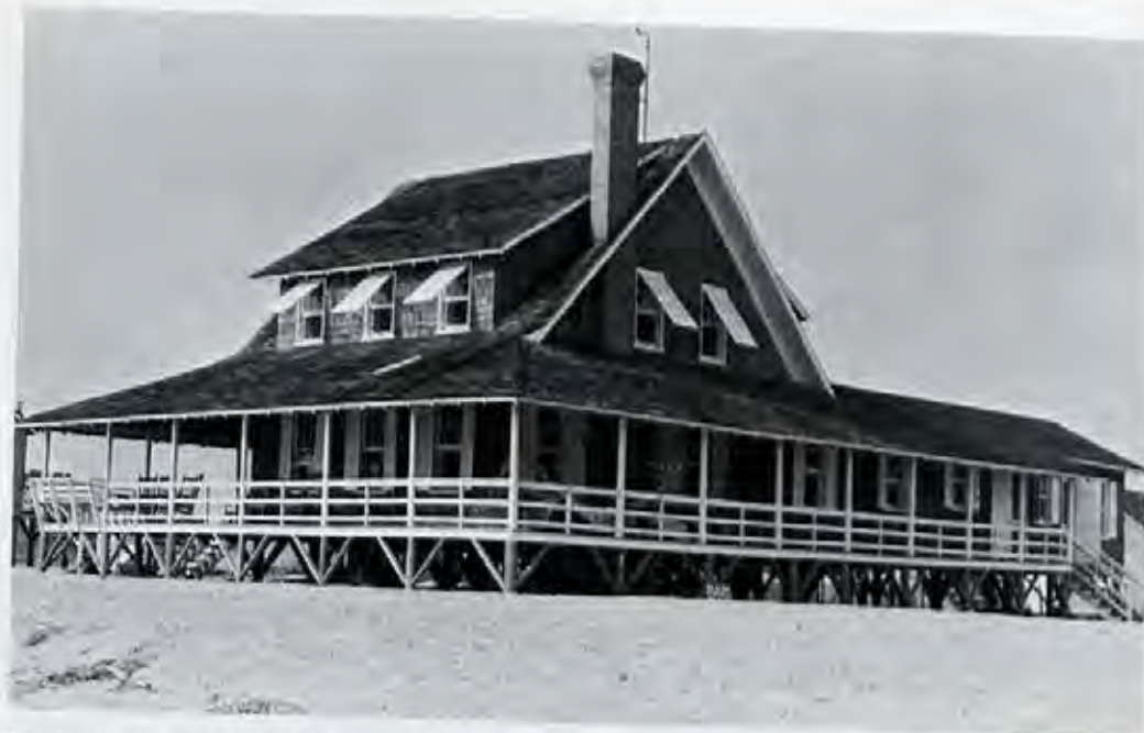
Figure 5. A large bungalow cottage with nearly full-width dormers, the most common house type in the Nags Head Beach Cottage Row Historic District.
