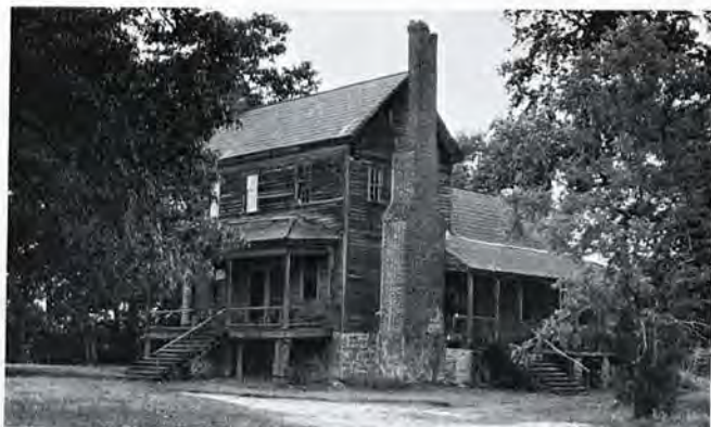
Figure 3. McLemore-Canady House, Franklin County, late eighteenth century. With the raised foundation and steeply pitched roof, the facade of this house is so vertical in proportion as to be a rectangle set on end. Here the builder showed no concern for the symmetrical placement of windows and doors. Each room of the hall-and-parlor first floor has a separate entrance. Note the massive, double-shoulder chimney; the shoulders are paved smooth. The roof has been rebuilt to extend over the gable ends.
