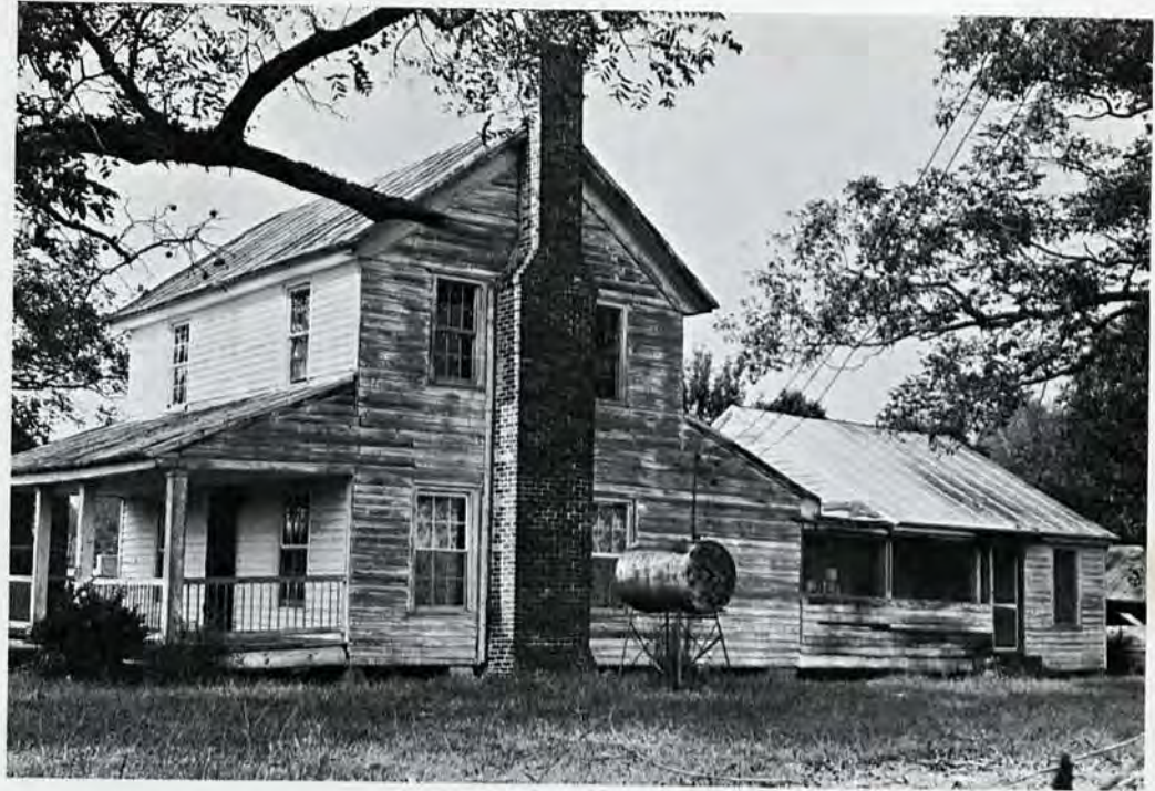
Figure 16. Two-story hall-and-parlor plan house with shed rooms, in Duplin County (also considered an I-house since it is two stories).
