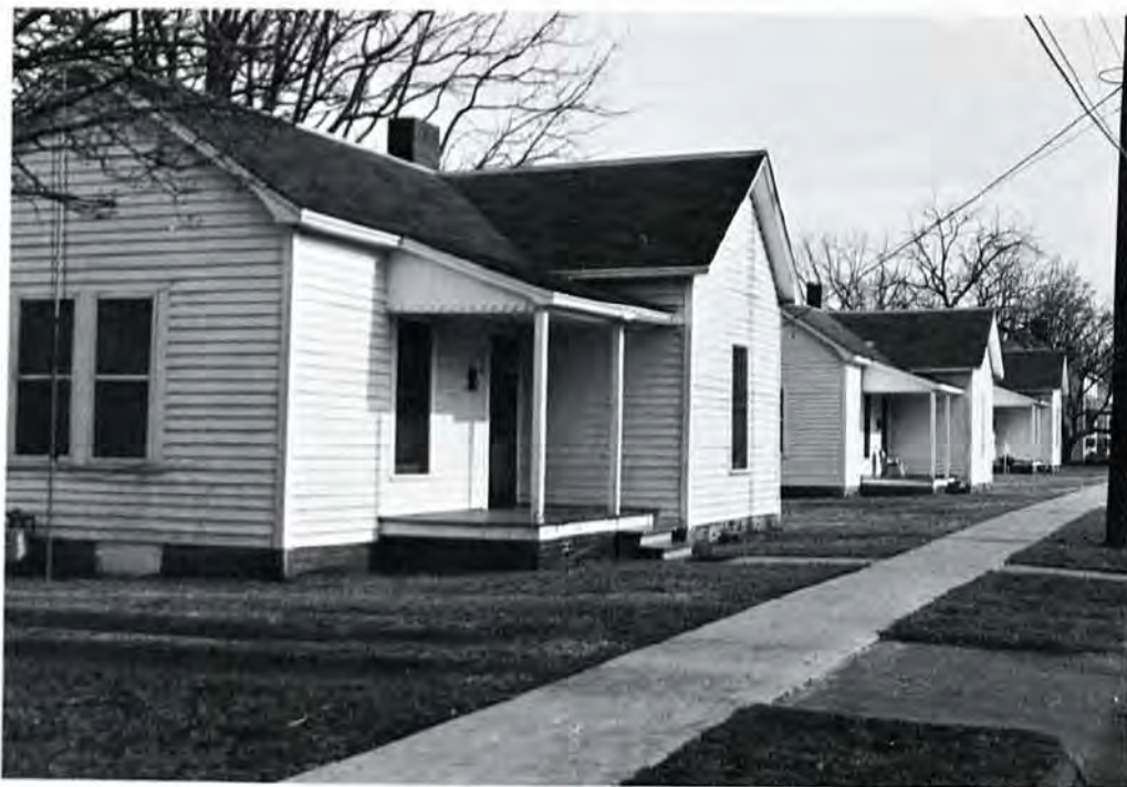
Well-maintained "company houses" in China Grove.
