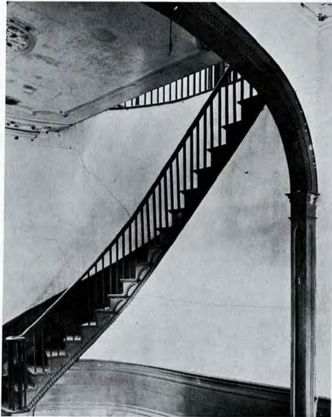
Figure 7. Prospect Hill. The graceful stair, while not freestanding as at Montmorenci, featured the same delicate scroll brackets on the treads, plus an interlaced guilloche molding.
