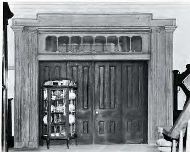
Figure 12. View of four-panel door which closes off one arm of the wide cruciform hall of the Buckner Hill House, Duplin County.
