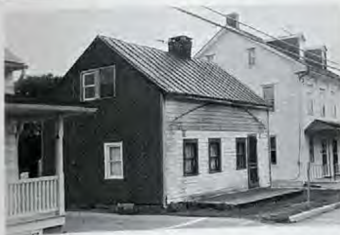
Figure 6. Continental plan log house, Newmanstown, Berks County, Pennsylvania. Similar small scale hall-kitchen plan houses comprise a significant portion of eighteenth century village architecture in other nearby towns such as Kleinfeltersville and Schaeffertown.
