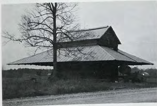
Cantilevered shed near Tabor City.
