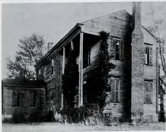
Figure 5. Prospect Hill, Halifax County. Many of the details of the exterior of Montmorenci are seen again at Prospect Hill, a house also dismantled. Door and window details are similar, and the porch, roofline, and cornerpost treatments are characteristic of the related houses.
