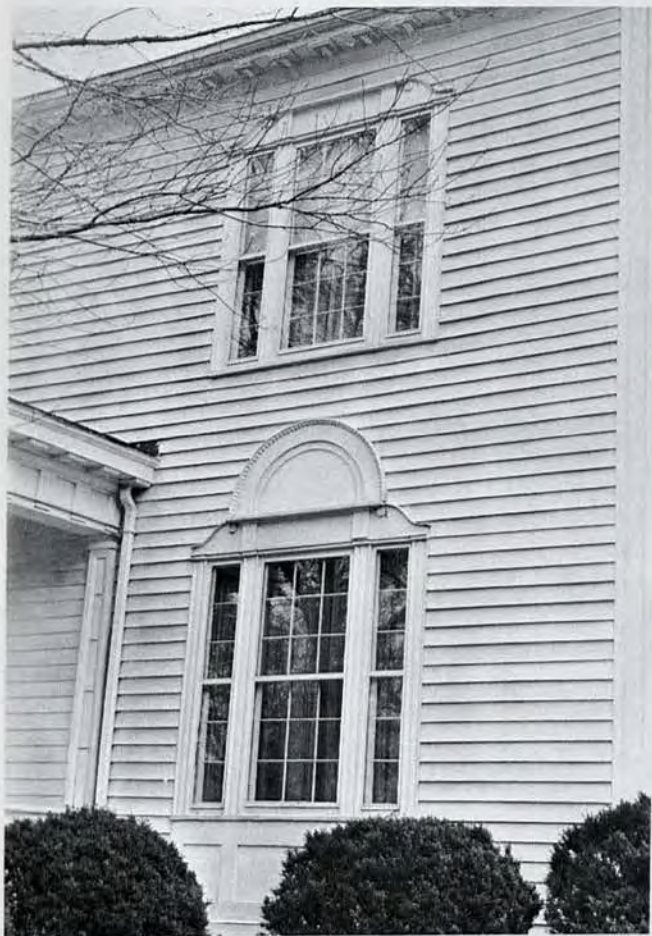
Figure 9. Coleman-White House, Warrenton. The detail of the windows is slightly simpler than at Prospect Hill and Montmorenci, but the treatment is essentially the same.
