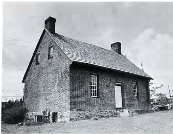
Figure 2. John Haley House, 1786. This extensively "restored" museum house was probably the largest and certainly the most substantial dwelling of its day in Guilford County.
