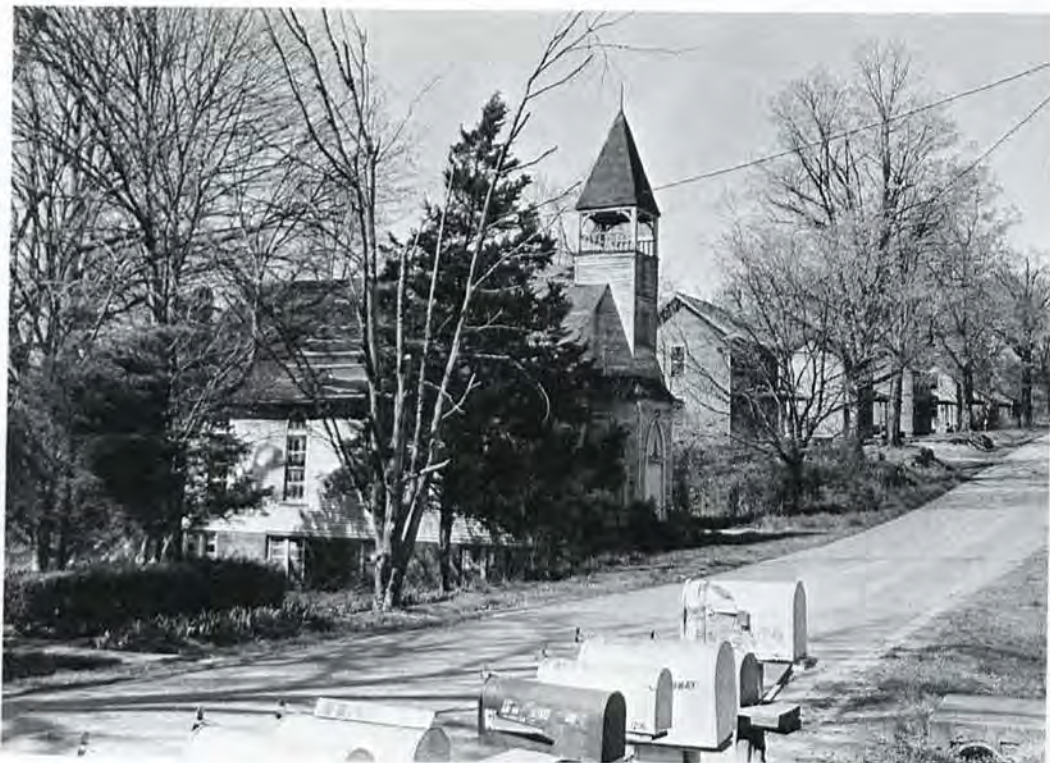
A recent view along one of Glencoe's residential lanes (prior to winter 1976 when the church roof collapsed).
