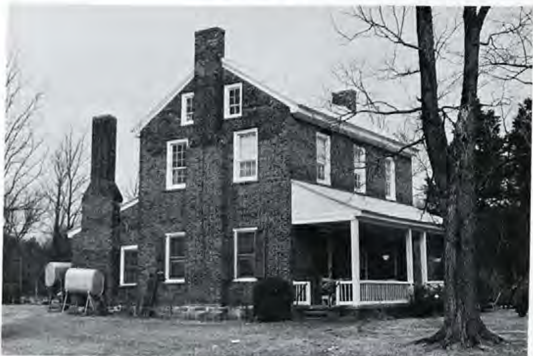
Figure 20. John Cowan House, vicinity of Bear Poplar, Rowan County, North Carolina, built about 1820. This later house is a good example of the Continental plan made regular and given a more fashionable symmetrical three-bay facade.
