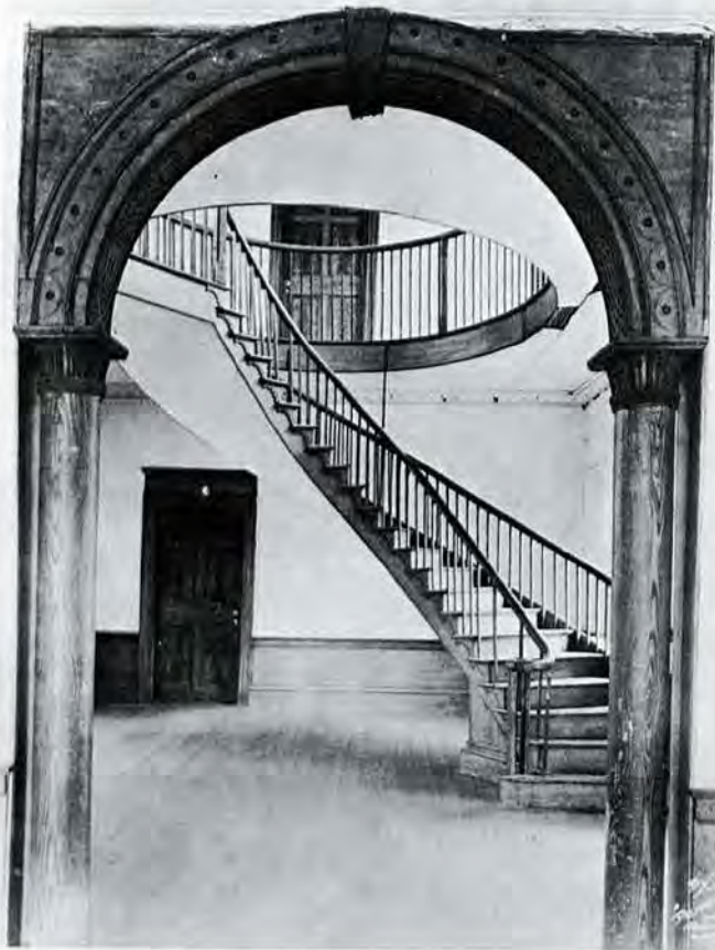
Figure 4. Montmorenci, stair, in situ . The elegant spiral stair was constructed in a trial-and-error fashion, recreating the grandeur of some of the finest houses of the eastern seaboard. A modified replica of the stair, with a different curve, was installed at Winterthur. The carved detail of the treads is repeated in other regional houses.
