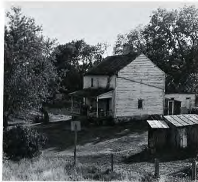
Figure 8. Continental plan log house, vicinity of Fischer's Hill Shenandoah County, Virginia. This dwelling displays the characteristics of the three-room plan house as found in Germanic-settled areas of Pennsylvania. The one-story rear ell is also of log construction.
