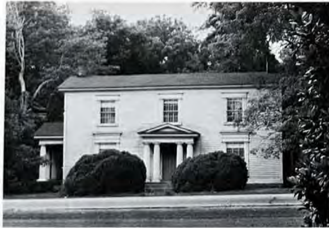
Figure 11. Shubal Coffin House, remodelled to present appearance ca. 1840. This plain center-hall plan house was vigorously treated on its facade with Greek Revival detail, the most elaborate surviving in the county. Despite its obvious crudity by academic standards, its owner consciously strove for the latest stylistic image.
