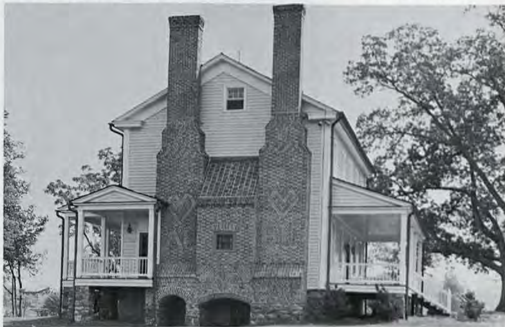
Figure 15. Alexander Long House, vicinity of Salisbury, Rowan County, North Carolina, showing patterned exterior end chimneys bearing initials and hearts.
