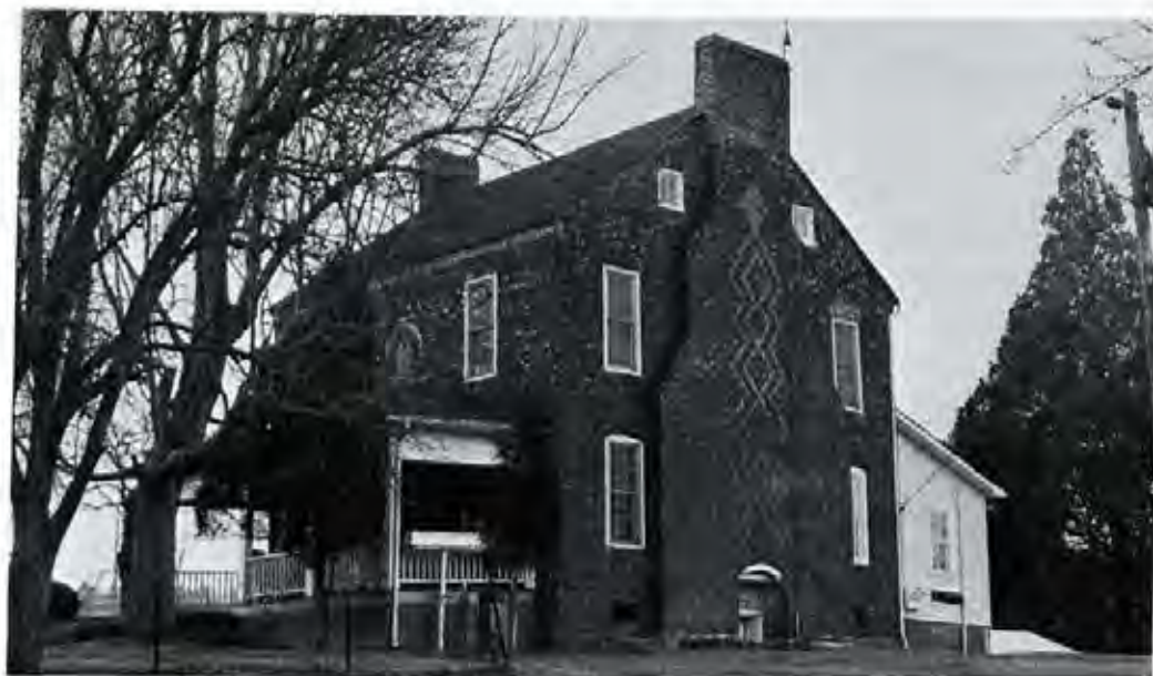
Figure 13. John Stigerwalt House, gable end showing patterned brickwork.
