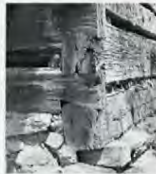
Corner timbering on barns in Caswell County: (top) V-notch, (middle) square, and (bottom) half dovetail.
