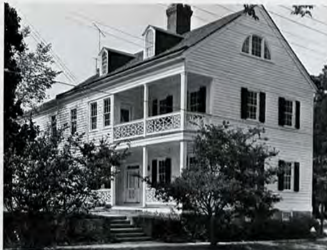
Figure 6. Coor-Gaston House, New Bern, ca. 1767, with porch finished like an interior room.
