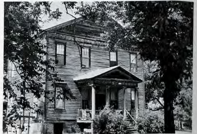
Figure 12. Dalkeith, Warren County. The temple-form house with characteristic cornice treatment; the porch is of a more typically classical character. The four-bay width and simply treated entrance are unusual.
