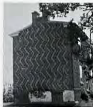
Figure 14. Chambliss House, Salem County, New Jersey, built mid-eighteenth century, altered mid-nineteenth century.
