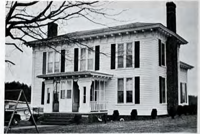
Figure 12. Ingle-Kraus-Hodge House, ca. 1850. In addition to its remarkable porch, the house contains a range of stylistic elements, including Italianate and Greek Revival motifs.
