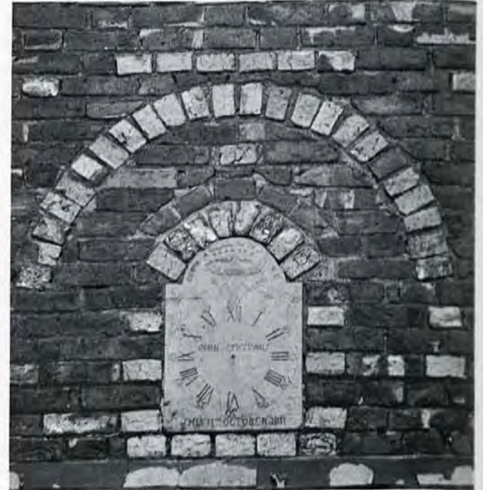
Figure 17. Stigerwalt House, detail of inset stone sundial framed by glazed header arch.
