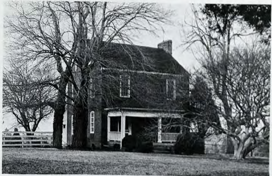
Figure 1. John Stigerwalt House, Rowan County, North Carolina, built about 1811.
