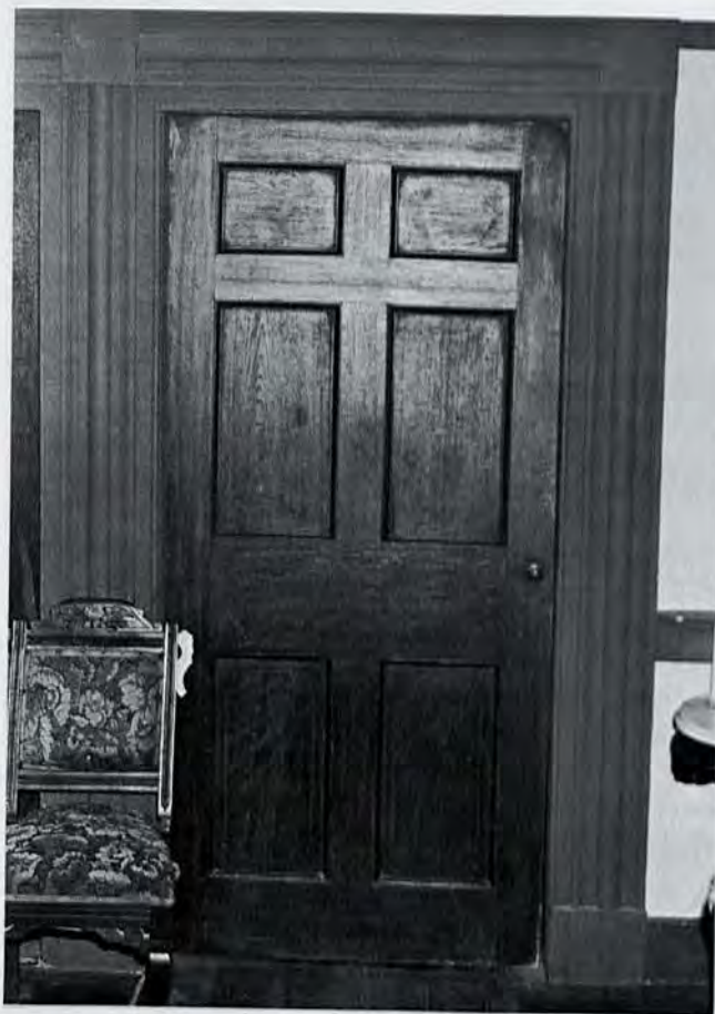
Figure 6. Charles Benbow House. Interior detail shows typical painted and grained Federal style door with painted inlay set in a robust and fully developed Greek Revival surround.
