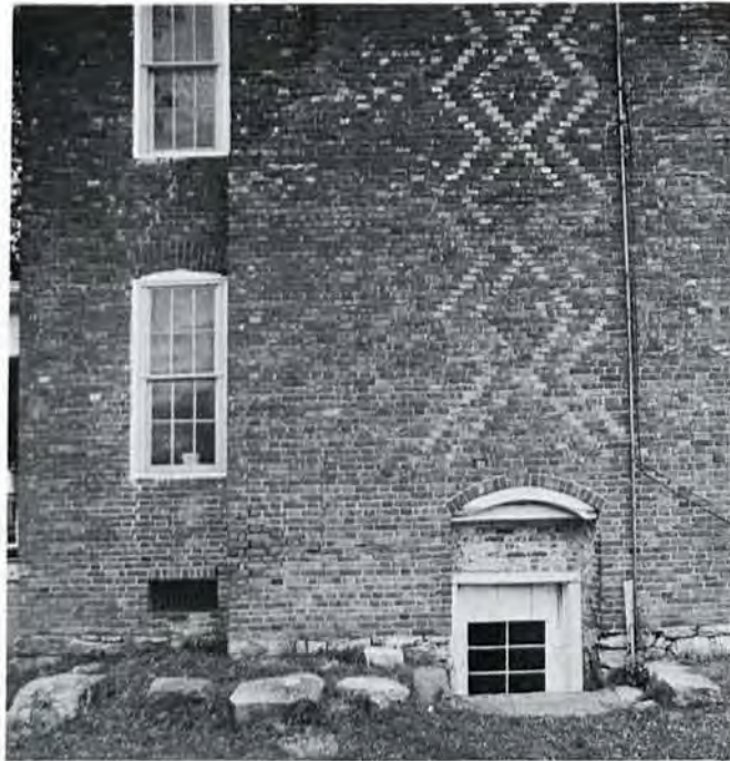
Figure 16. Stigerwalt House, detail of lozenge work in the east gable end.
