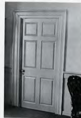
Figure 7. Georgian-type door. Six raised panels in a three-part surround.
