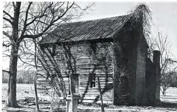
Figure 19. Matthias Phifer Log House, vicinity of Third Creek Church, Rowan County, North Carolina, built about 1806. This small Continental plan dwelling displays a transitional two-bay second floor, three-bay ground floor combination. The shed element with independent chimney is original and common in the locale.
