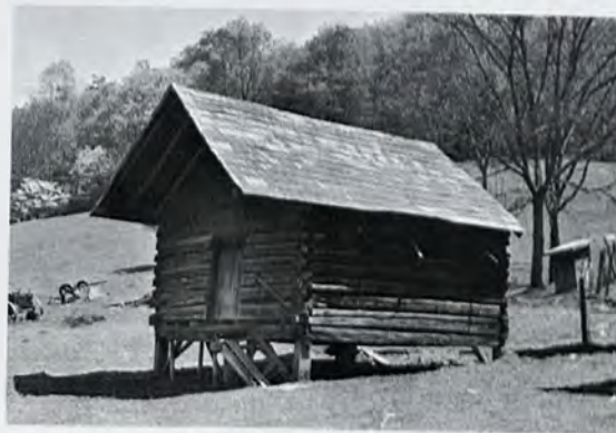
Figure 15. A log granary on the Alex Woodruff Farm, Alleghany County. Built in the nineteenth century the granary is on raised wood piers to protect its contents from the nesting of rodents. As is frequently seen on log smokehouses the roof is extended on the front gable end to shelter the entrance.
