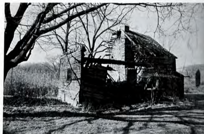
Figure 4. Pott Log House, vicinity of Lobachsville, Berks County, Pennsylvania, built mid-eighteenth century. In ruins, the Pott House provides a rare cross section of the formal features of a Continental plan house including a two, rather than three, room plan and large central fireplace.
