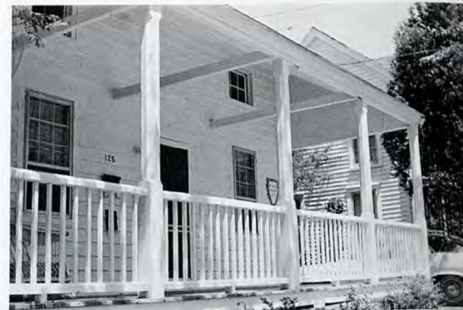
Figure 13. Attic ventilation window above the ceiling joists of the Jesse Piver House porch in Beaufort.
