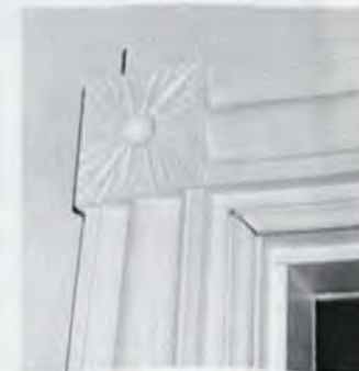
Figure 10. Low House, located in the heart of Guilford's German settlement. Interior detail shows Greek Revival style door surround with unusually treated corner block. Other details are fully developed Federal style.
