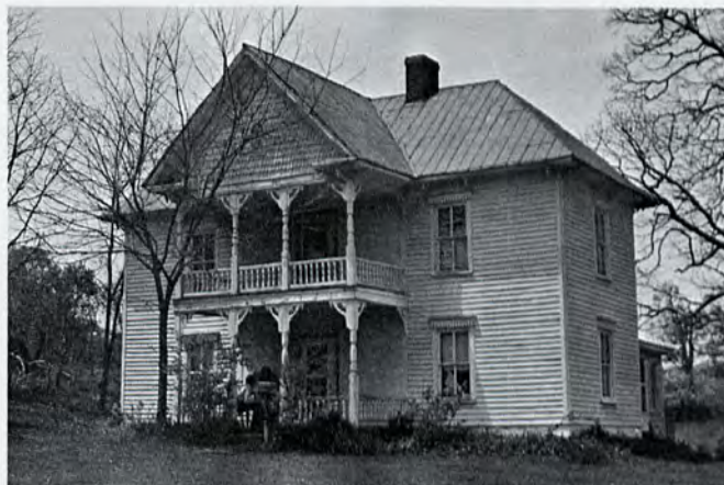
Figure 10. The William H. Billings House, Alleghany County. The use of decorative woodwork is seen here at its best on the two-story pedimented porch which with the other ornament under the eaves and on the window surrounds transforms this otherwise simple and typical frame house into the seat of a prosperous landowner and businessman.
