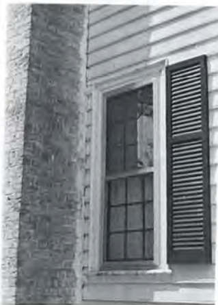
Figure 5. Georgian-type window. Nine-over-nine sash, three-part molded and mitred frame, and molded window sill. Note beaded weatherboard.
