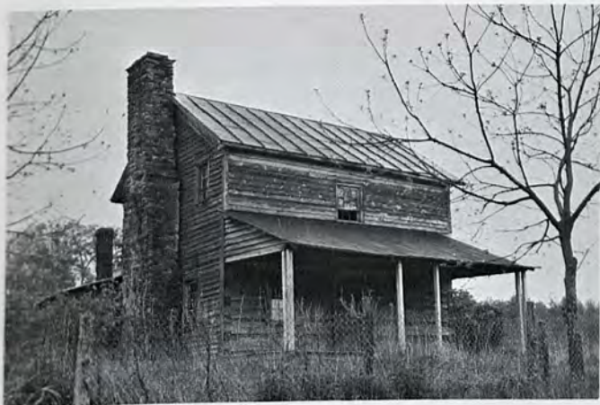
Figure 2. The Samuel Cox House, Ashe County. This full two-story log house is typical of the second generation of log building in the valley. The log construction of this house is visible under the shed porch where the weatherboards have been removed. The form of the porch is original to construction while its roof and supports have been replaced.
