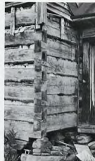
Figure 3. The Samuel Cox House, Ashe County. The full dovetail joints of the log construction are well illustrated here where the weatherboards have been removed.
