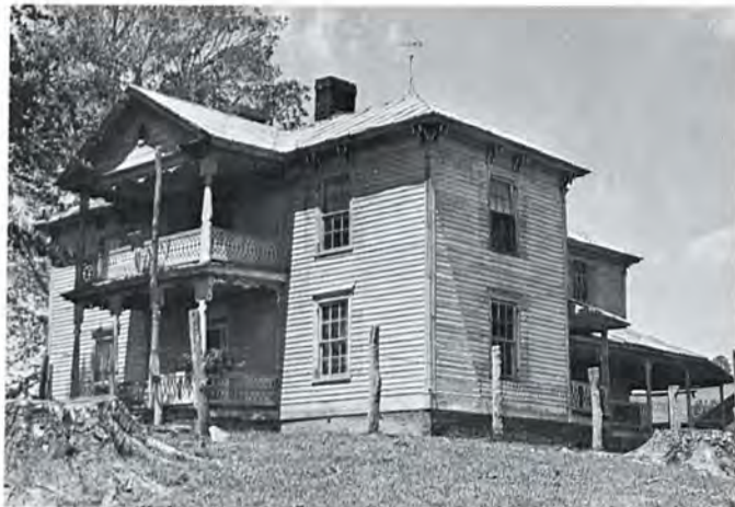
Figure 12. The John F. Greer House, Ashe County. One of the largest and most ambitious of the late-nineteenth century frame houses in the valley, this seat of the important Greer family has richly ornamented front and rear porches while the eaves are supported by paired brackets set above the fenestration and at the corners of the house.
